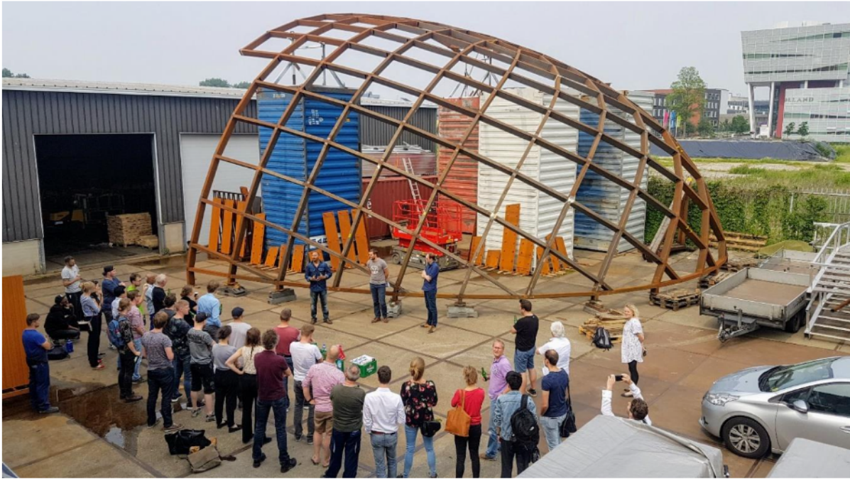
Fig. 13 Test-assembly steel pre-assembled frames.
